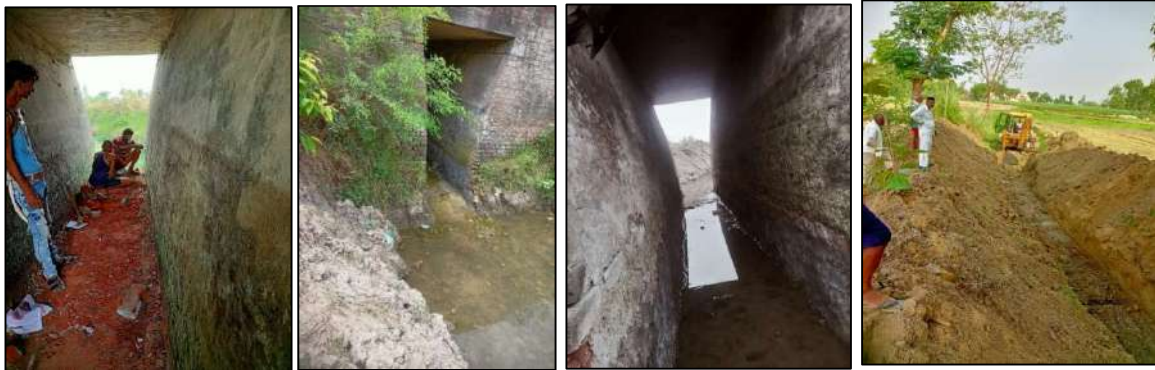
Fig 2. Construction of drainage channel with convergence irrigation department
